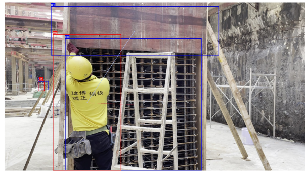
Figure 3. Installing formwork [16]
